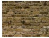
London stock brick - English bond Used on rear and side facades
