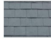
Natural slate roof Used on front mansard roof
